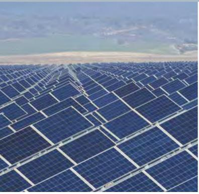
Solar panels on solar tracking systems automatically track the position of the sun to yield maximum energy depending on the time of the year and the length of the day.
